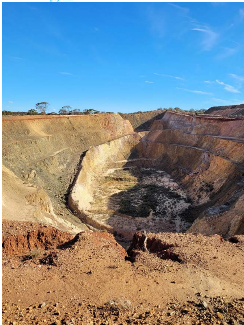
Figure 18 Big Blow Mine Pit showing no indication of water
