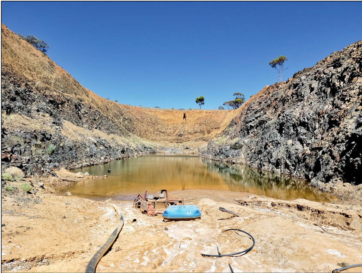
Figure CNX Existing Pit with Shallow Water
