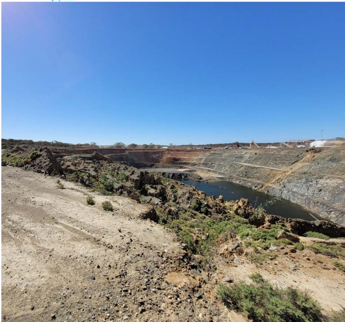
Figure 14 Greenfields Pit showing water in pit and slumping of Pit Wall on Northern Side
